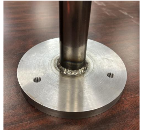
Figure 5: Picture of TIG-weld between mounting plate and tower.
